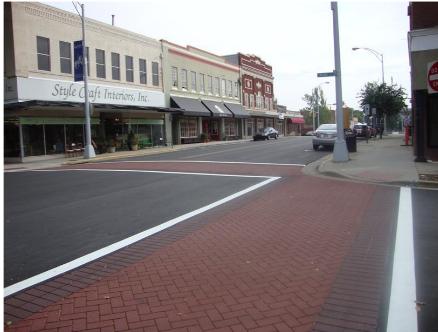
StreetPrint Textured Asphalt Crosswalk, NC
