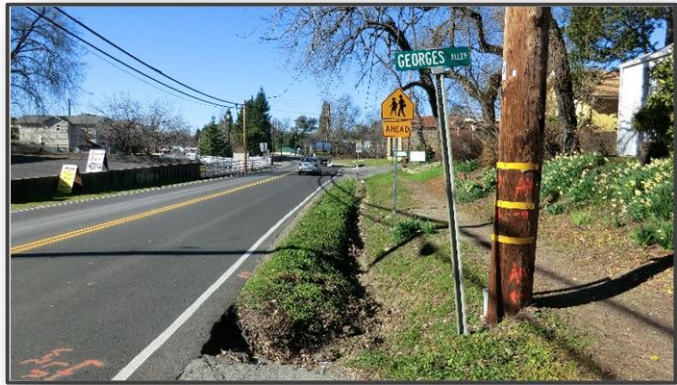
Worn pedestrian path on Pleasant Valley Road
