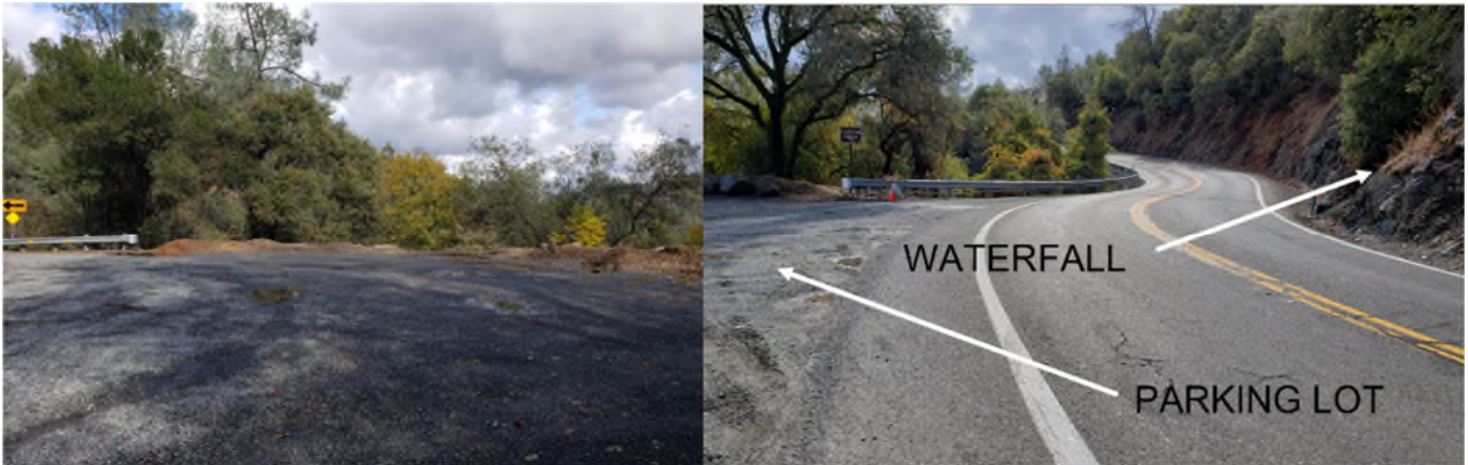
FIGURE 4343: PHOTO OF SR 49 AT CANYON CREEK EASTBOUND
