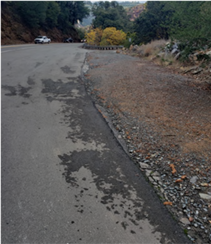
FIGURE 5252: PHOTO OF SR 49 PARKING NEAR PM 35.5 EASTBOUND
