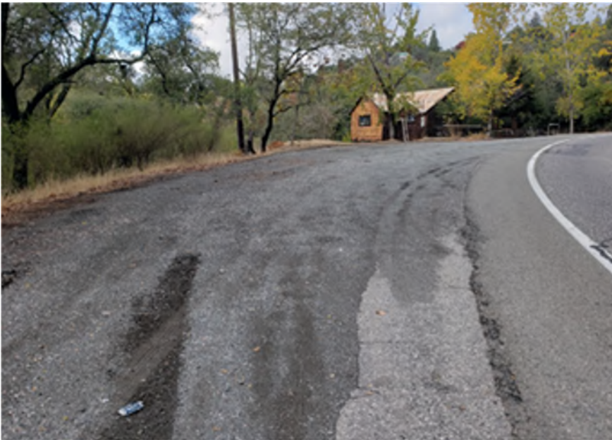
FIGURE 3838: PHOTO OF SR 49 NEAR PM 2.0 EASTBOUND
