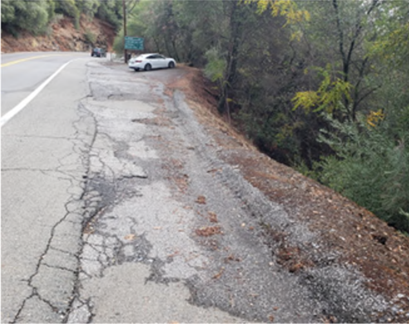
FIGURE 3737: PHOTO OF SR 49 PULLOUT AREA NEAR PM 2.15 HEADING EASTBOUND
