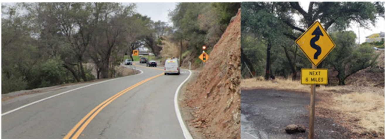
FIGURE 3636: PHOTO OF SR 49 NEAR LINCOLN WAY SIGNAL (LEFT - WESTBOUND, RIGHT - EASTBOUND)
