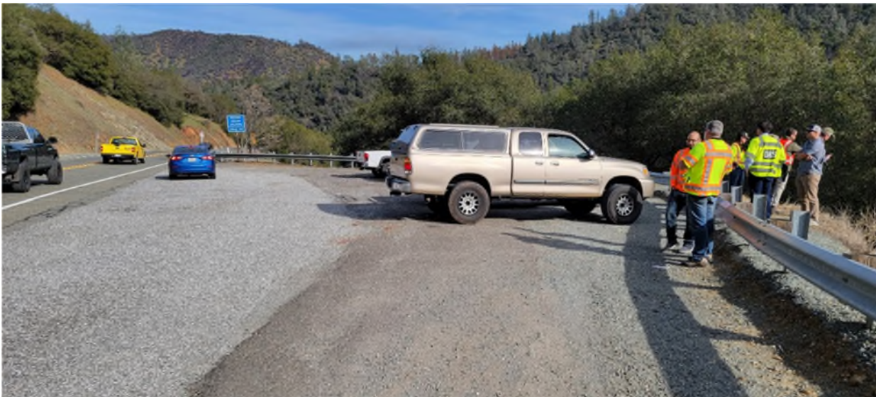
FIGURE 4444: PHOTO OF SR 49 NEAR PM 0.7 EASTBOUND
