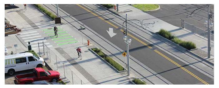
Intersection crossing markings can be used at signalized intersections or high volume minor street and driveway crossings.
