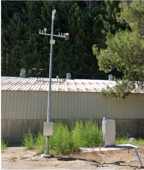
FIGURE 33. CALTRANS ITS STATION WITH TRAFFIC AND WEATHER SENSORS ON US 50 WEST OF ICE HOUSE ROAD
