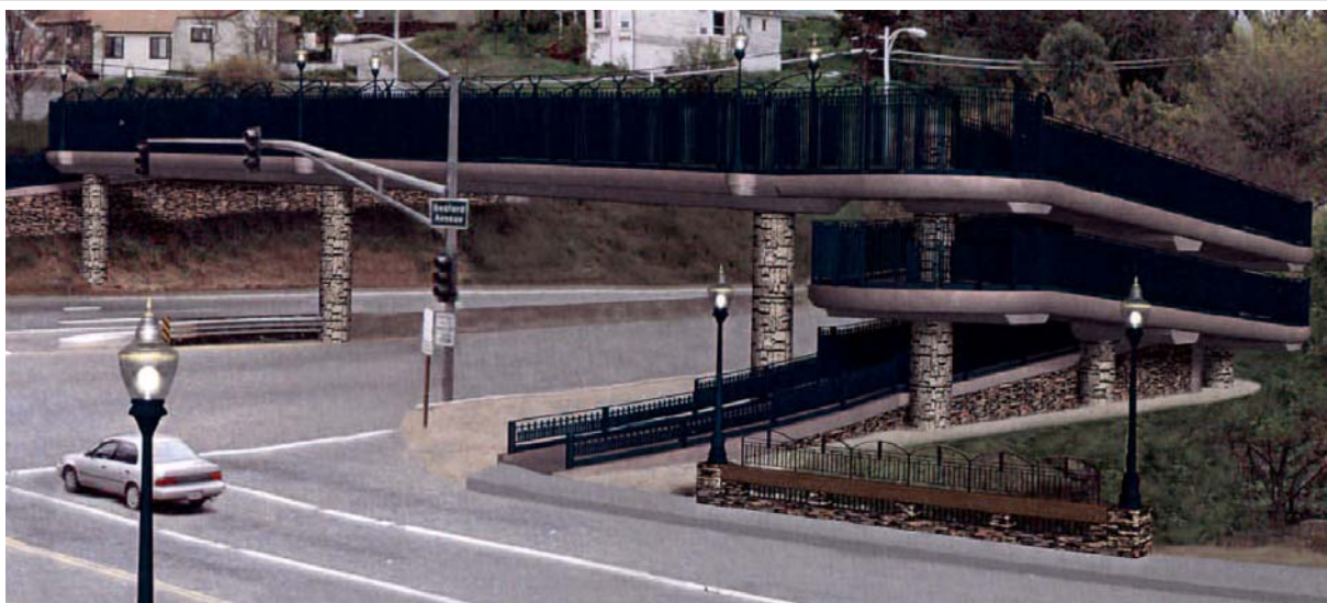
Caltrans photo simulation of Bedford Pedestrian Overcrossing to be constructed as a component of the Highway 50 Operational Improvements project.
